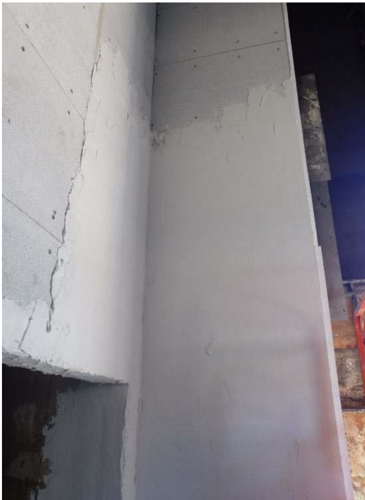
FIGURE 6: CEMENT RENDER INSTALLATION
