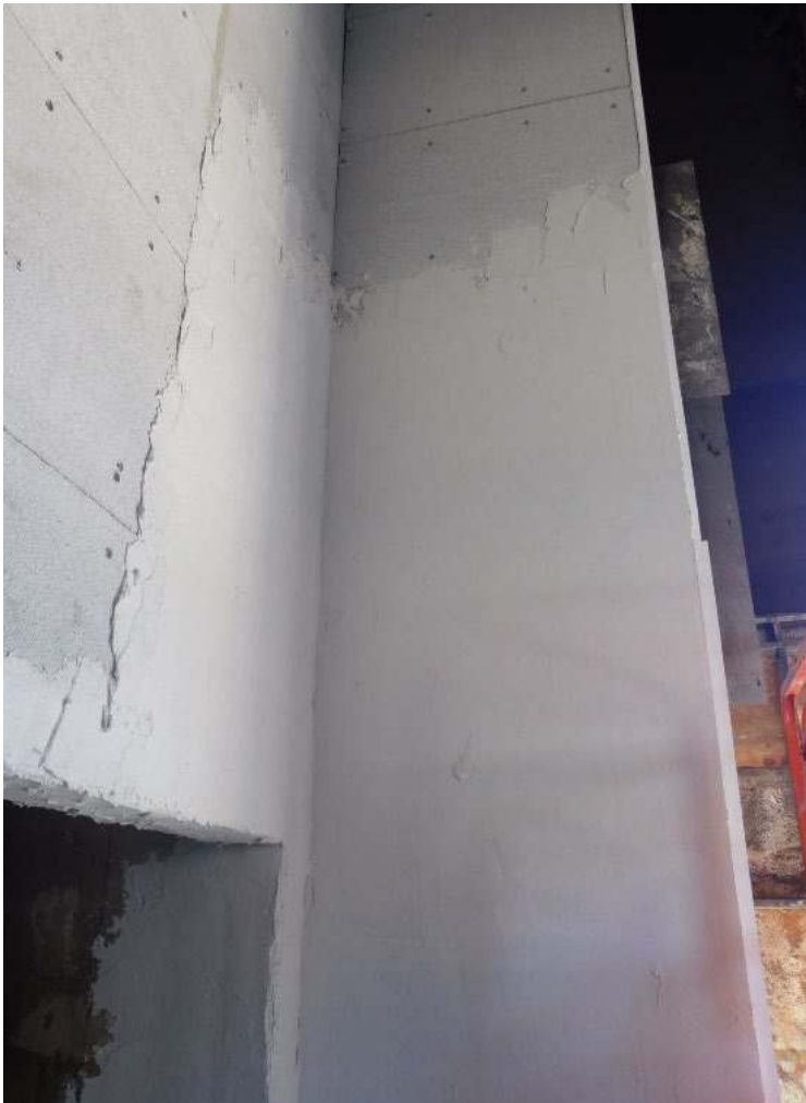
FIGURE 6: CEMENT RENDER INSTALLATION
